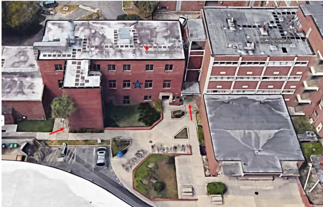
Figure. A 3D view of Dr. Broadbent's office (blue star) and two entrances (red arrows) to access the '3rd' floor. The office door is located directly across from the Geomatics administrator's main office.
